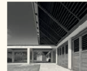
Detail of roof vents at Reef House, Vanuatu, used to capture prevailing sea breezes and cross-ventilate the house.
