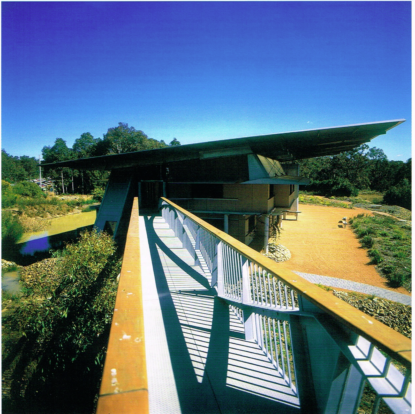
02. Looking back from the footbridge reveals a spectacular double-roof, providing a void over ceiling for thermal control. KJ
